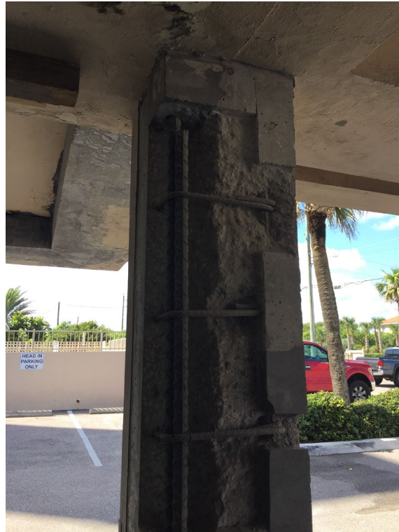
Picture 1: Approved column excavation
